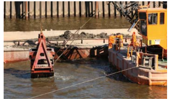
Harbour construction with sheet pile walls
