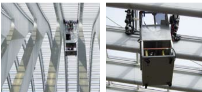
Service cart in vertiginous heights
